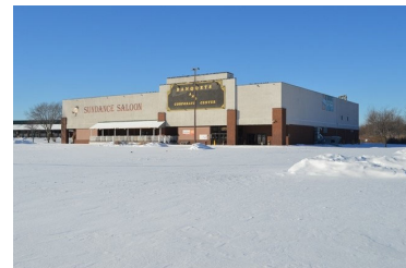
Waukegan Empty Retail $32.69 psf Deferred Maintenance
