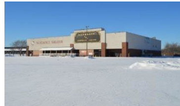
Waukegan Empty Retail $32.69 psf Deferred Maintenance
